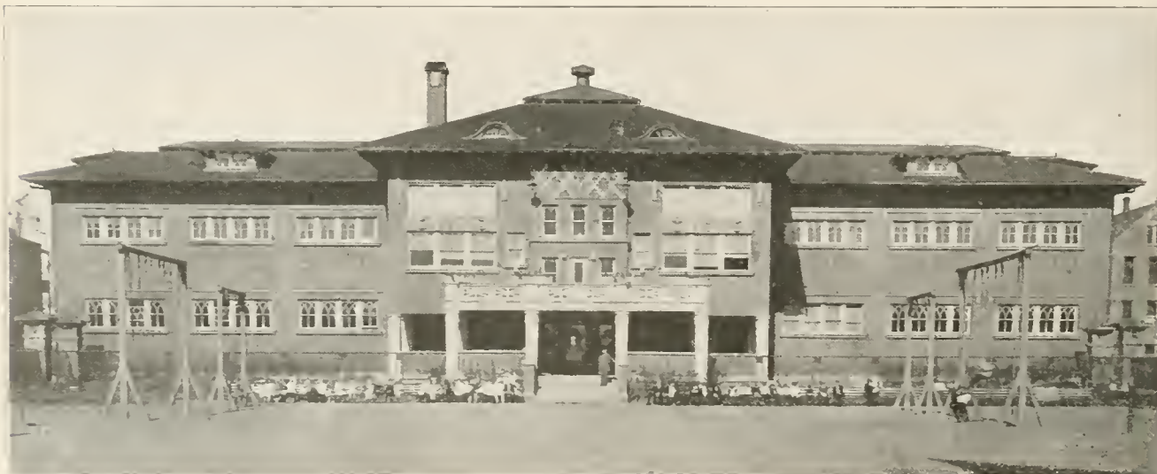
Holstein Park Recreation Center is a typical recreation plant. Millions of dollars have been spent throughout the country on community houses of this character. Few of them are being used to full capacity. The question is raised whether they could not be utilized more intensively for raising the health standards of their communities.
